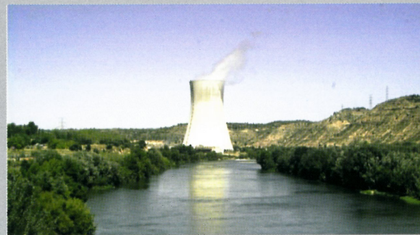
River Ebro as it passes by the Asco Nuclear Power Plant
