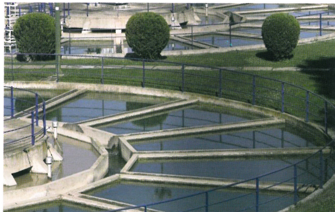
Drinkable water treatment plant in Zaragoza
