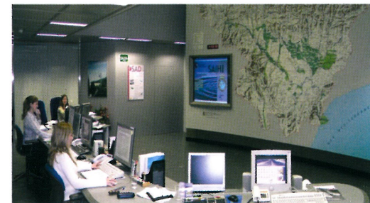
Point of control and measuring stations of the SAIH network.
