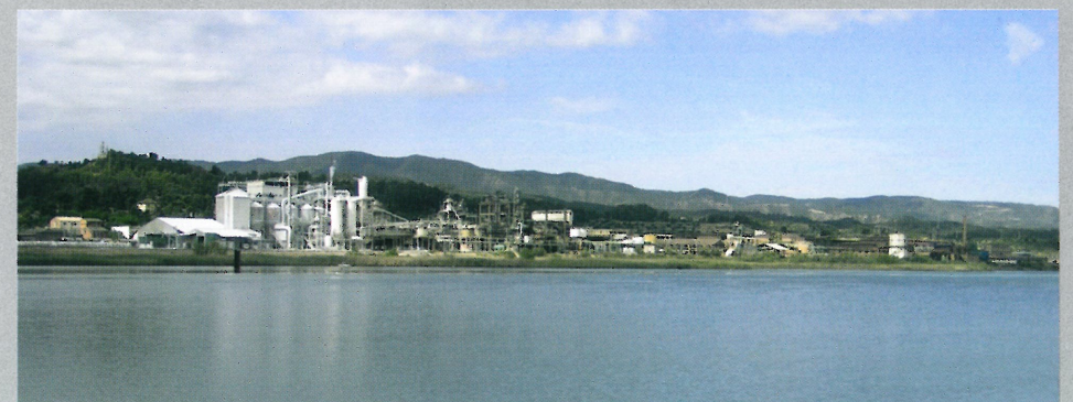
Work to remove sludge at the Flix reservoir
